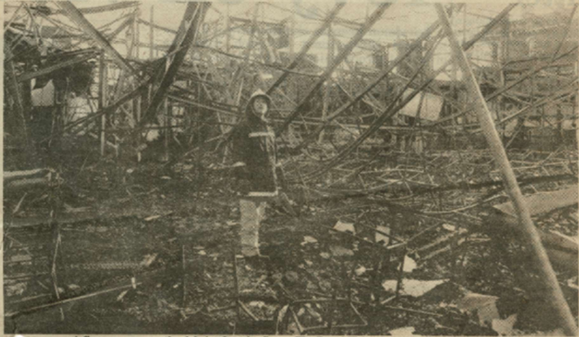
A fireman surveys the debris after the fire at The Royal Wolverhampton School
