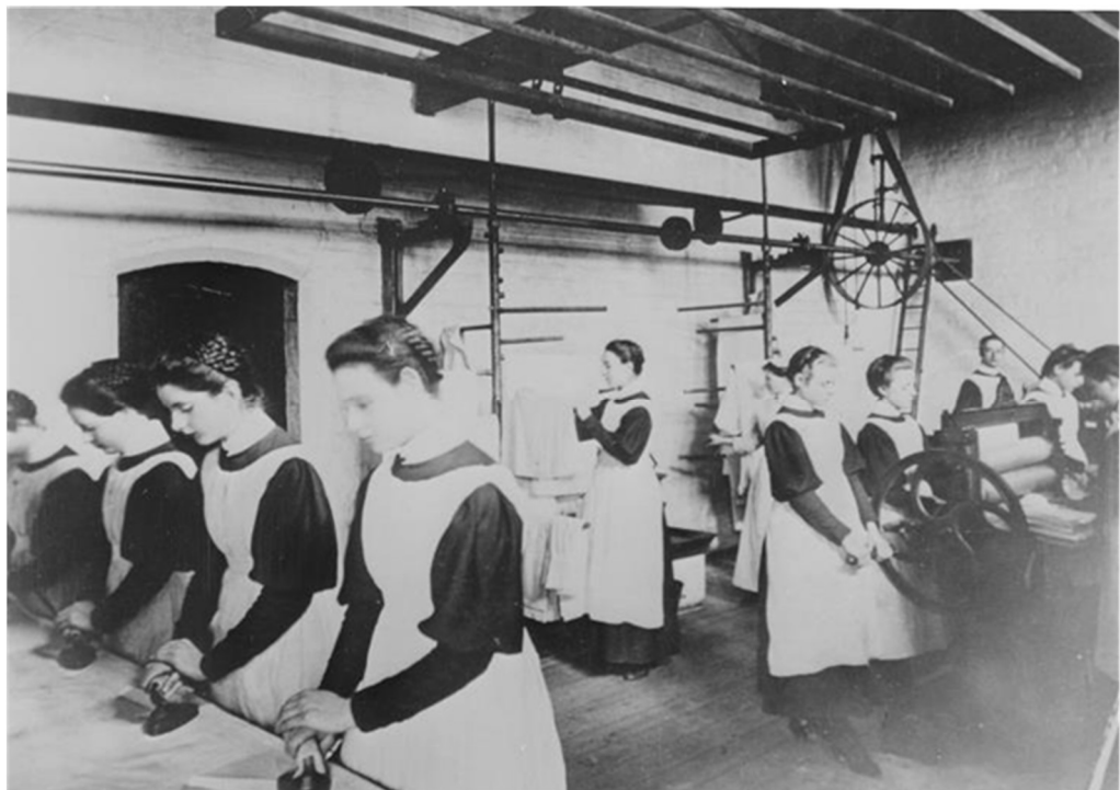
A laundry class. The girls are using flat irons, drying racks and mangles. This image also shows mechanical line shafts and pulleys, and empty overhead clothes drying racks.
